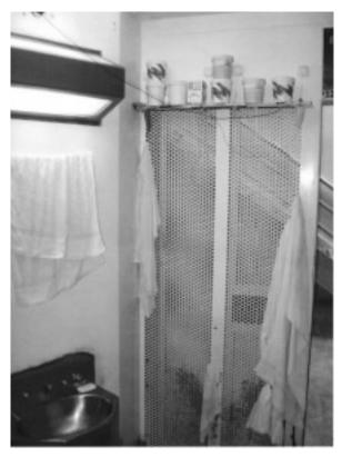
Front of a cell with perforated metal sheet, as viewed from inside cell<sup>29</sup>
